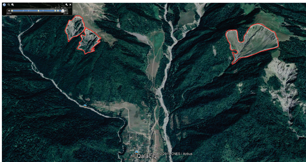
Fig. 7 Mudflows areas of the Goychay River basin and threatening the village of Galajig
