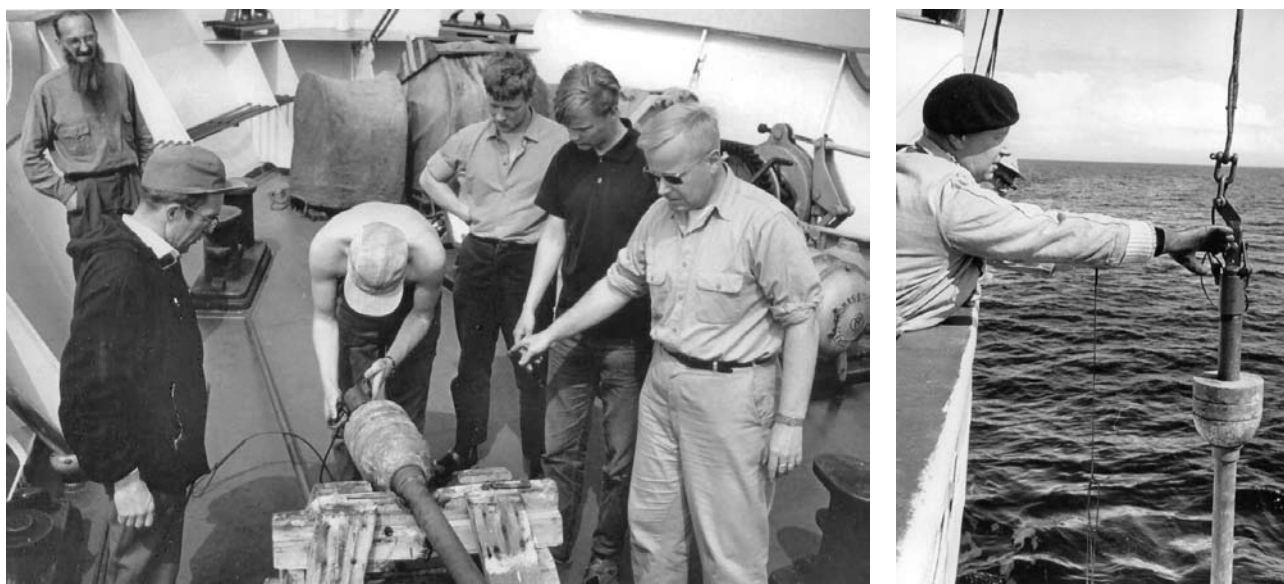
Fig. 1 The complexity of the original Kullenberg piston corer with 60 cm long brass core liners was already in 1964 exchanged into a more realistic easy to use version with 5 metre long PVC-plastic core liners and a simplified release mechanism. On board Aranda bearded FIMR chemist Svante Nordström watching in the background and observers crowding young geologist Esa Kukkonen working while Dr. Heikki Ignatius oversees the assembly of the corer (above) and demonstrates the new release mechanism (right)
